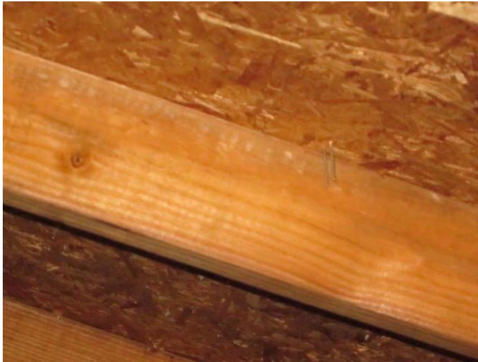
Roof Deck Attachment
