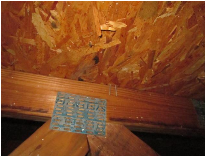
Roof Deck Attachment
