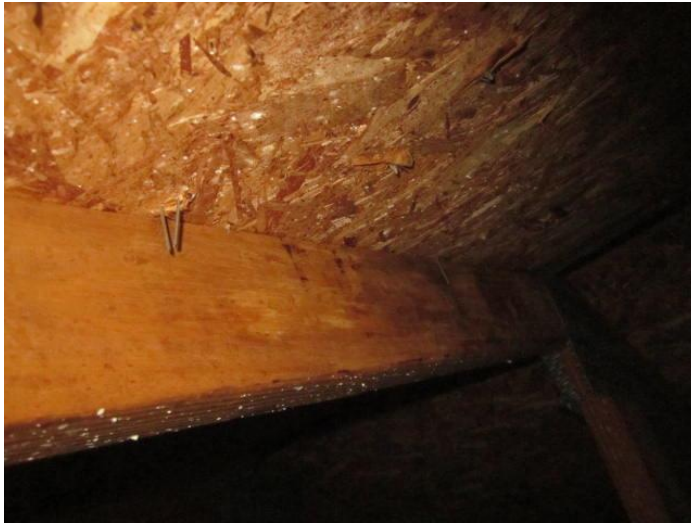
Roof Deck Attachment
