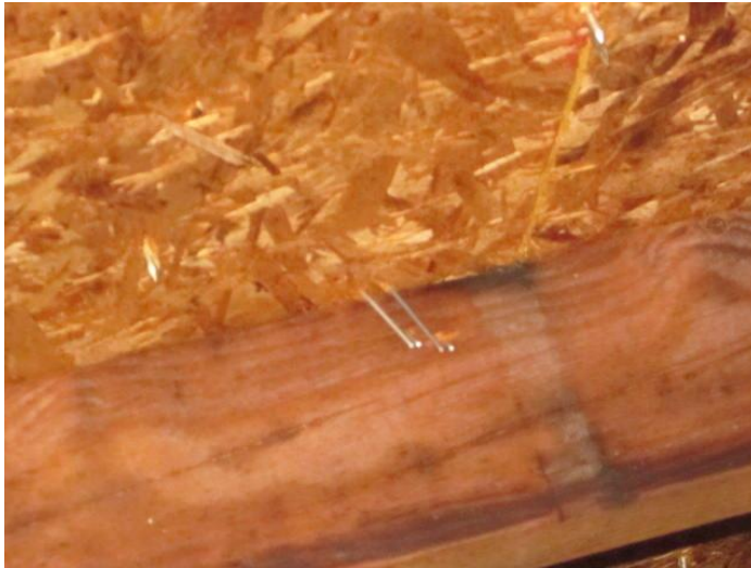
Roof Deck Attachment
