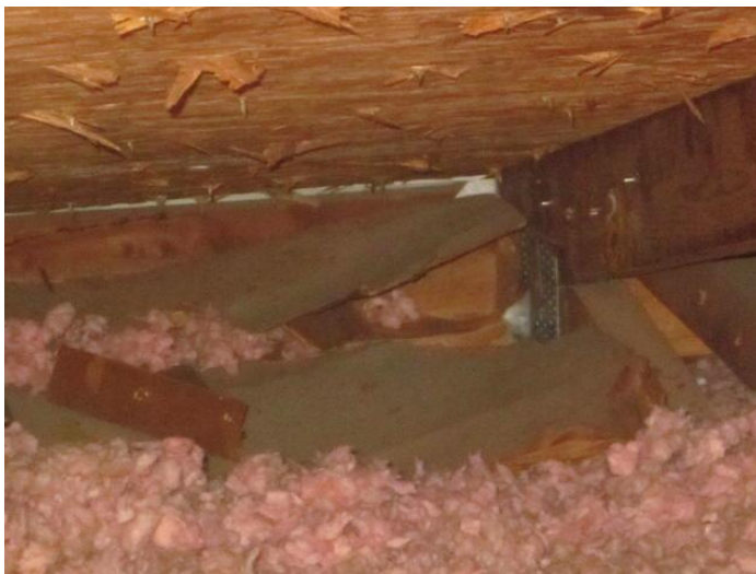
Roof to Wall Attachment
