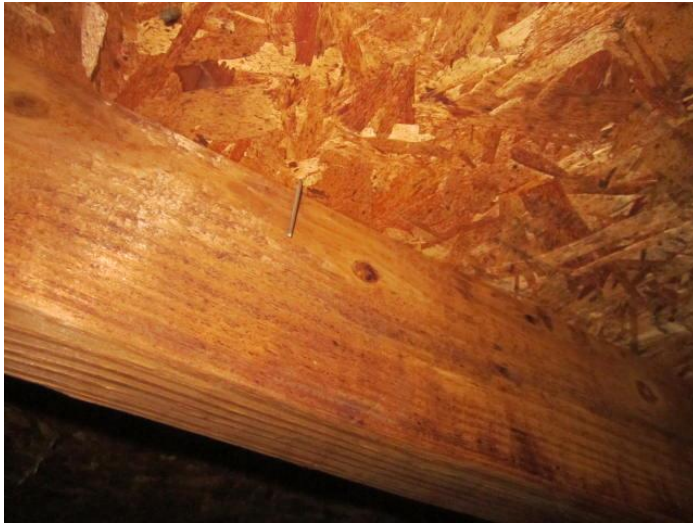
Roof Deck Attachment
