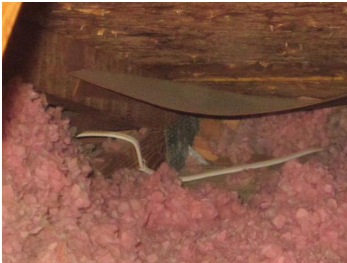
Roof to Wall Attachment
