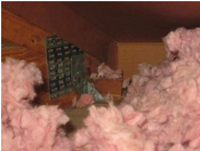
Roof to Wall Attachment
