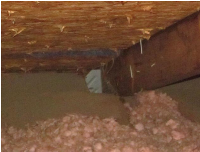
Roof to Wall Attachment
