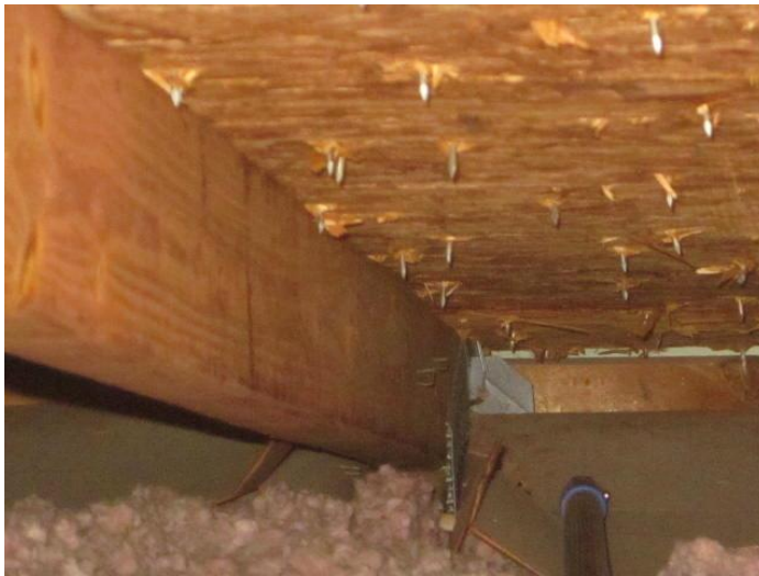
Roof to Wall Attachment
