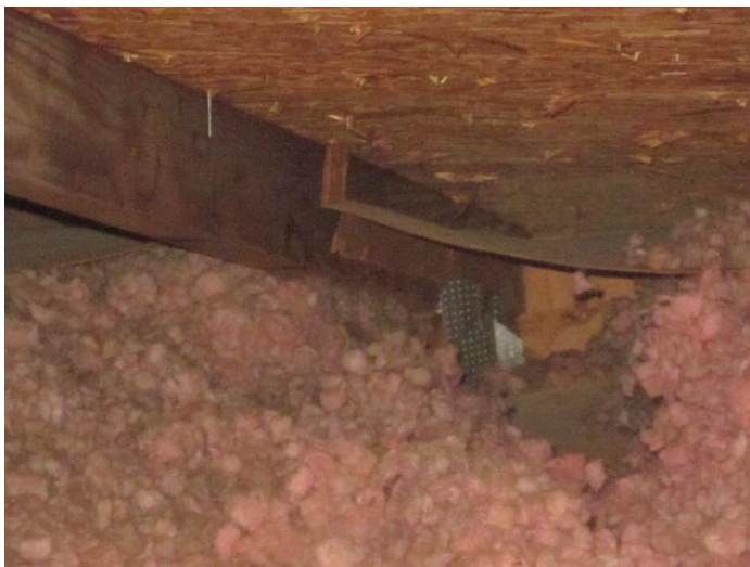
Roof to Wall Attachment
