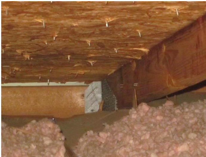
Roof to Wall Attachment
