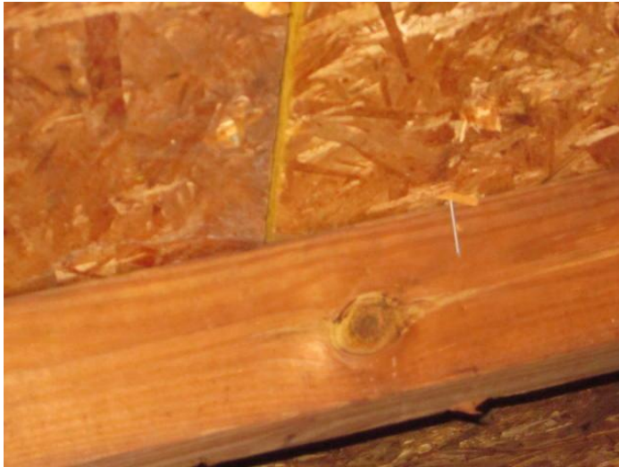
Roof Deck Attachment
