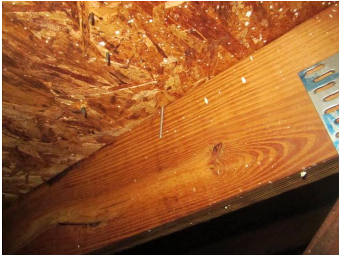
Roof Deck Attachment
