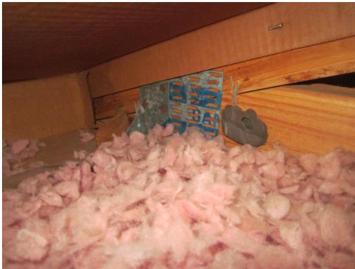
Roof to Wall Attachment
