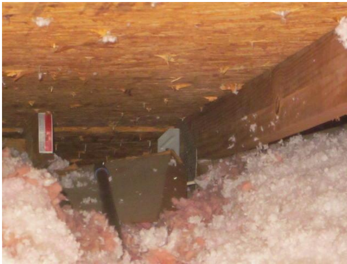
Roof to Wall Attachment
