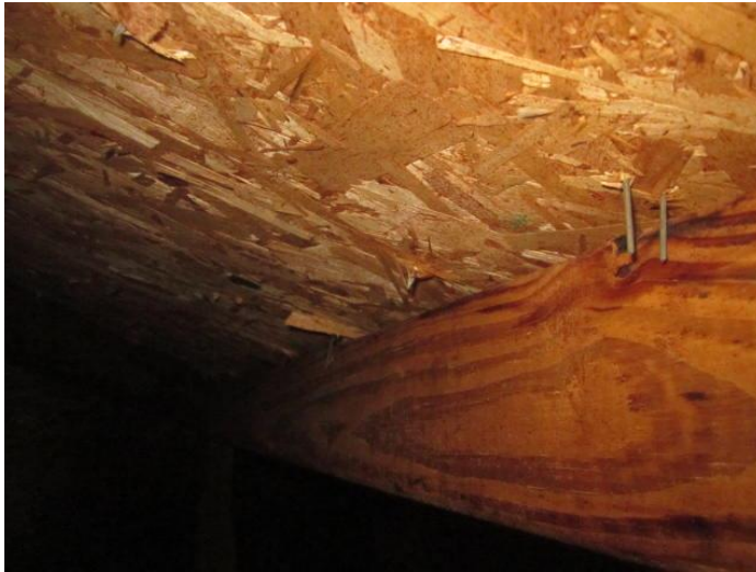
Roof Deck Attachment
