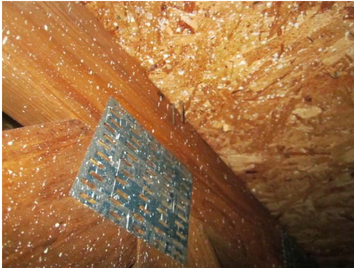
Roof Deck Attachment
