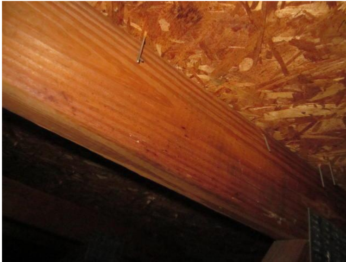
Roof Deck Attachment
