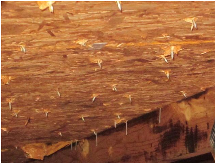
Roof Deck Attachment
