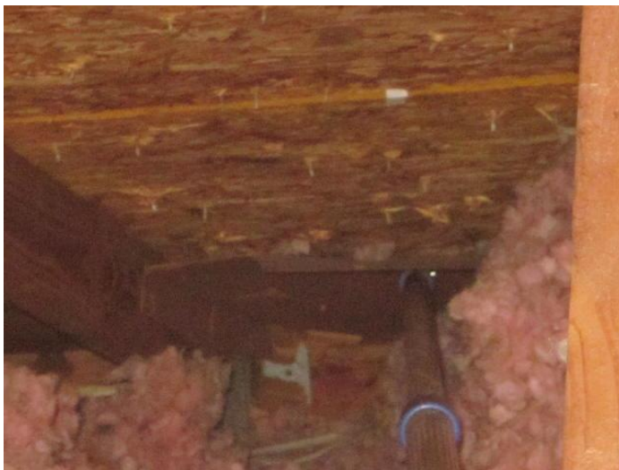
Roof to Wall Attachment
