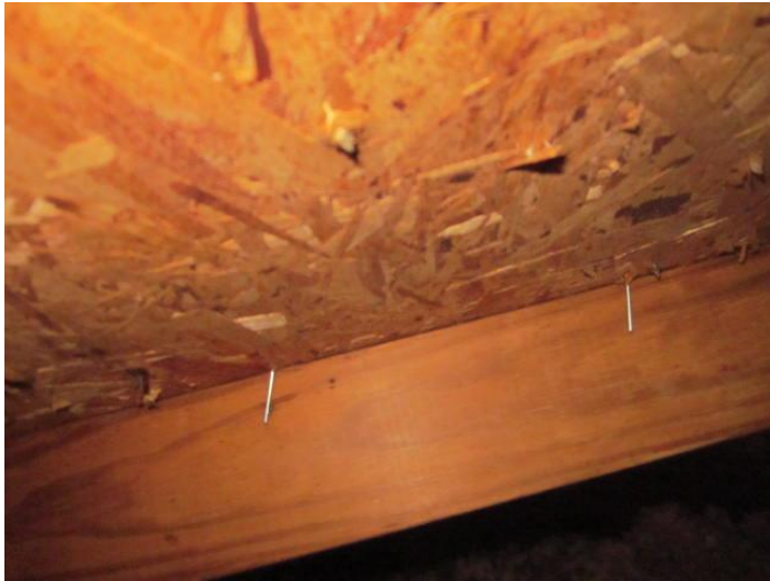
Roof Deck Attachment
