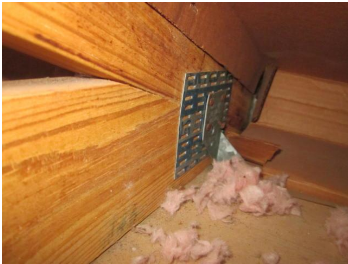
Roof to Wall Attachment
