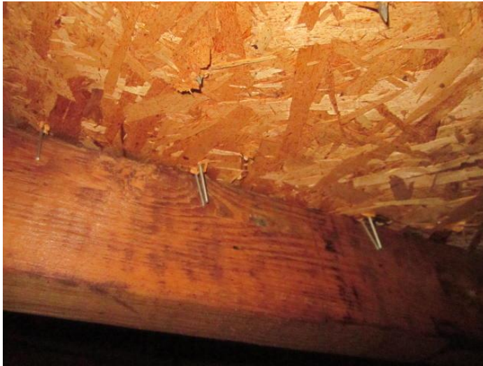
Roof Deck Attachment
