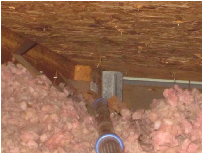
Roof to Wall Attachment
