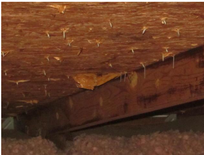
Roof to Wall Attachment
