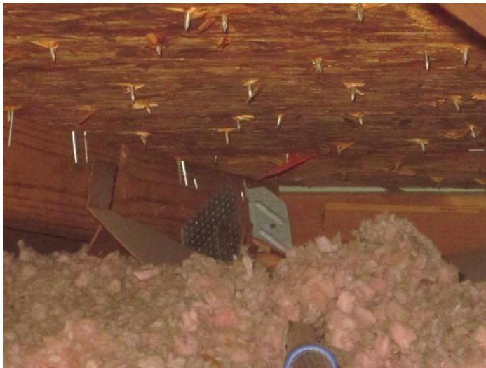
Roof to Wall Attachment
