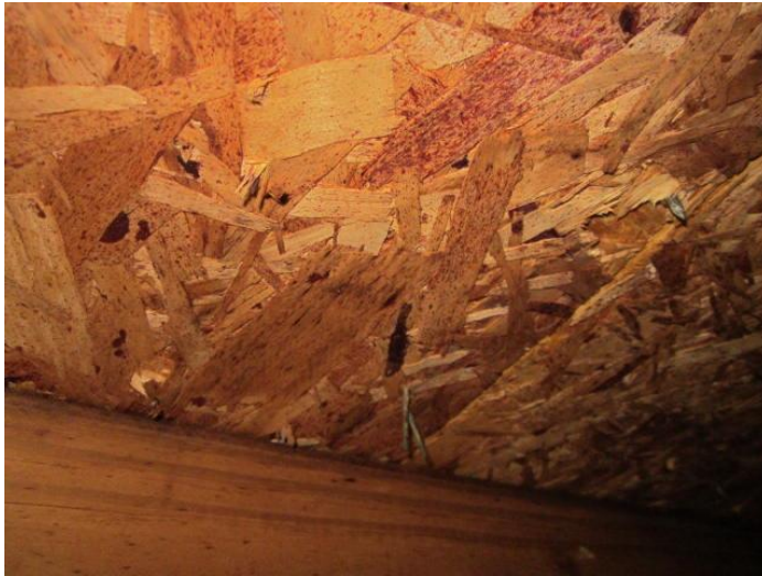
Roof Deck Attachment
