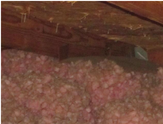
Roof to Wall Attachment
