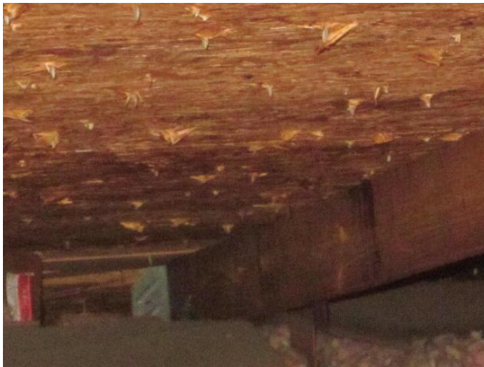
Roof to Wall Attachment
