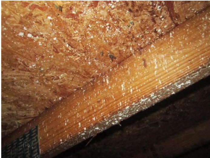
Roof Deck Attachment
