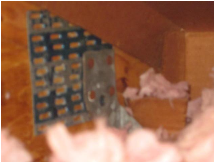
Roof to Wall Attachment
