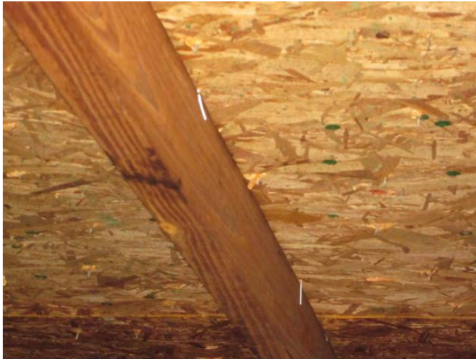
Roof Deck Attachment
