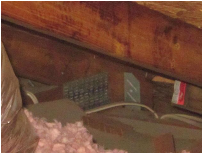
Roof to Wall Attachment
