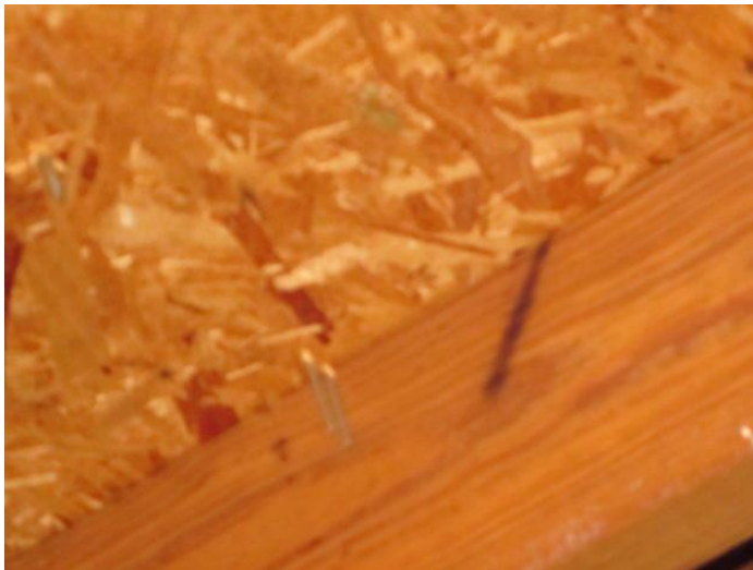
Roof Deck Attachment
